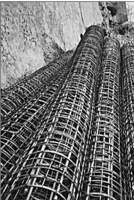
Preformed rebar for columns
