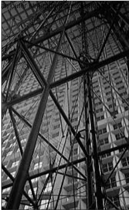
Tubular sections form the La Grande Arch structure in Paris.
