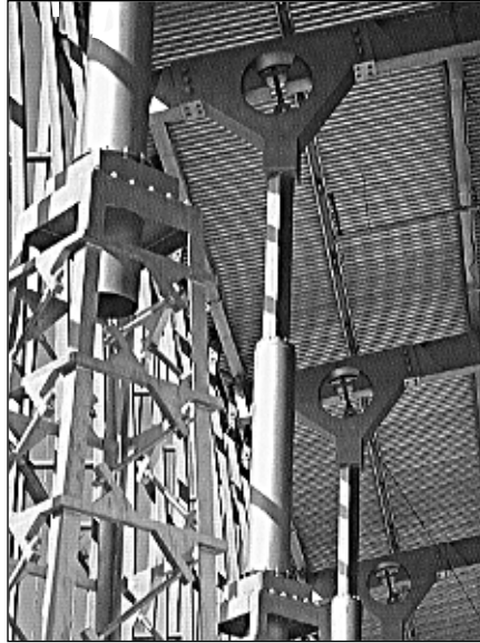
Tubular supports for the roof structure of the Canadian Archives Building.
