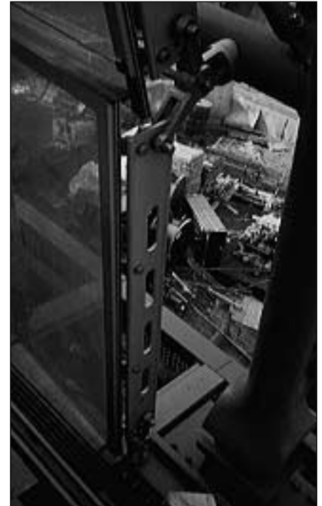
Complex stainless steel investment casting connecting the tubular structure with the glass wall.
