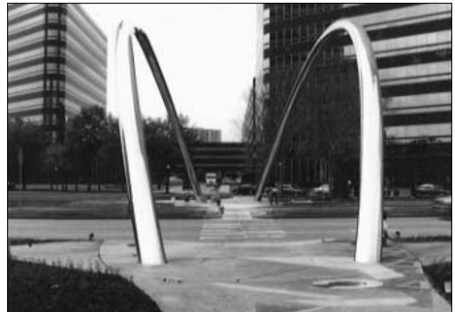
Arches, strut light covers and traffic signal poles (not in photo) were fabricated from 316L Stainless steel by the Offenhauser Company. The project is in the Galleria area in Houston.
