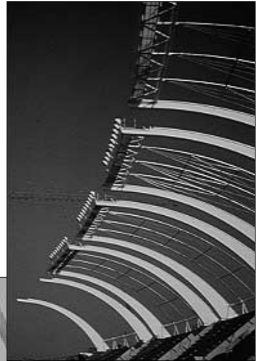
(photo, above) Stainless steel was used to support a lightweight PTFE coated glass fiber woven fabric roof (not yet installed).
