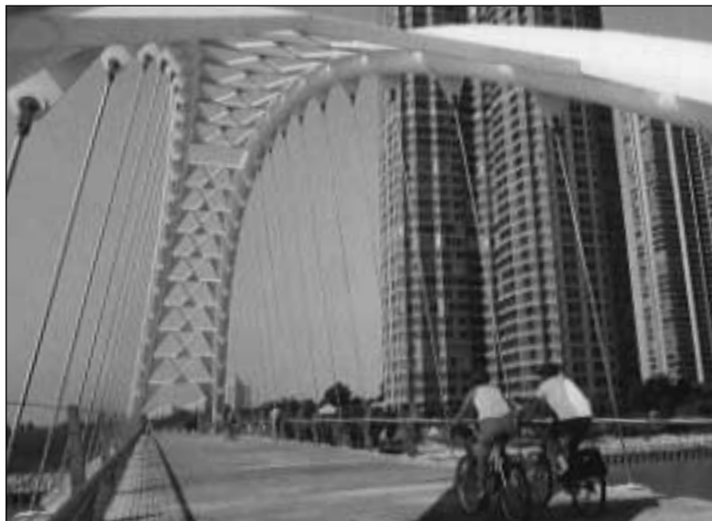
A continuous reinforced concrete slab supported by 44 stainless steel rods provides pedestrians and cyclists a bridge over the Humber River in Toronto.
