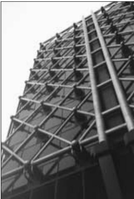
Structural tubes, filled with water, used as an external fire prevention system.
