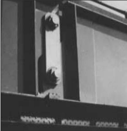
The Minnesota Department of Transportation replaced conventional low alloy steel with stainless steel hinge pins and hangers on the Blatnik Bridge in Duluth, Minnesota.
