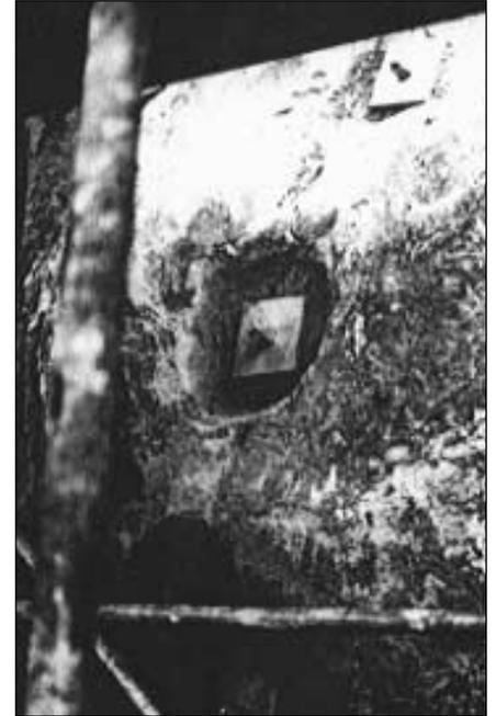
Lewis bolts (top) and threaded inserts for hanging stone (bottom) show variety of stainless steel fastening devices used in stone and concrete anchoring systems.
