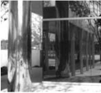
Stainless steel was used for the column covers and storefronts as well as the mullion cladding for the I.B.M. Building in Kansas City. The fabricator was Zahner Architectural Metals of Kansas City, Kansas.
