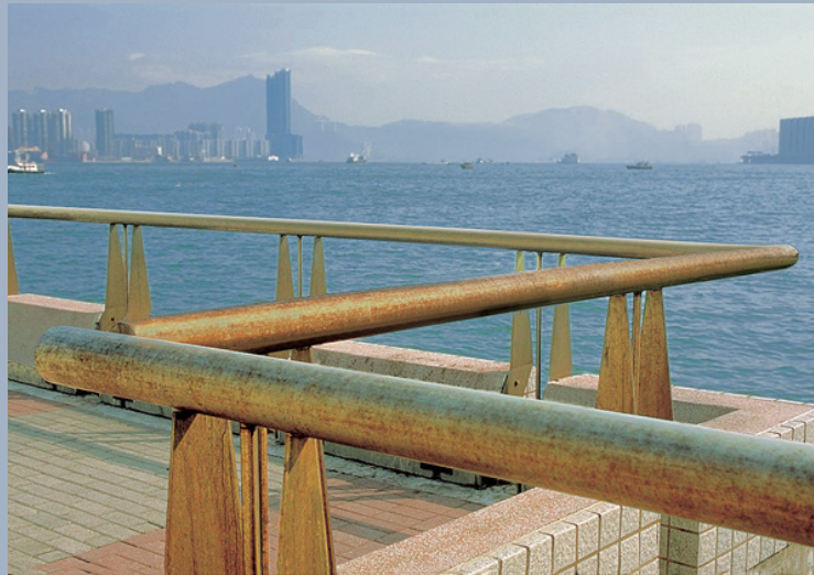
Hong Kong Convention Center railings, Type 316
