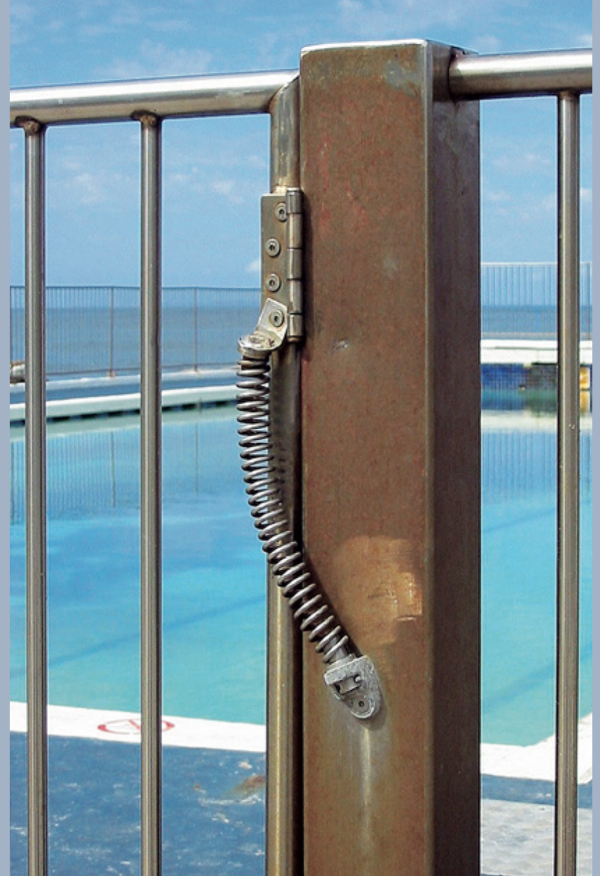
Australian Coastal fence, Type 316 gate and Type 304 post
