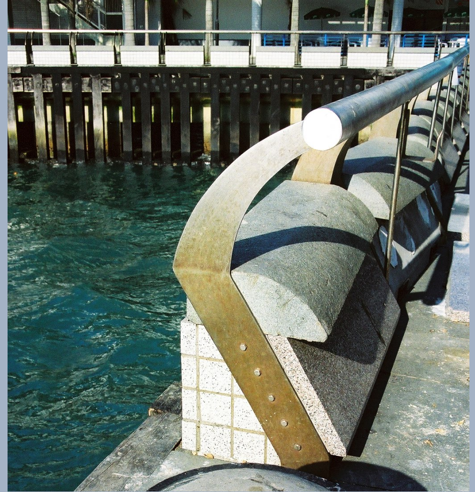
Type 316 railings Hong Kong Convention Center - seawater spray exposure, rough finish
