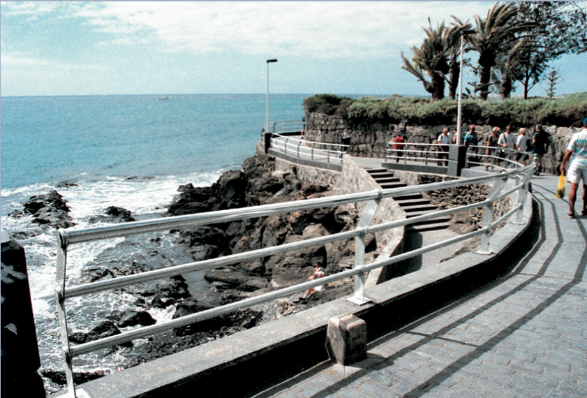
Canary Island railing, 2205 stainless steel
