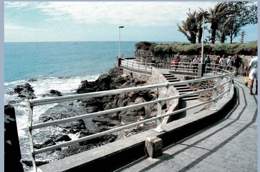
Canary Island railing, 2205 stainless steel
