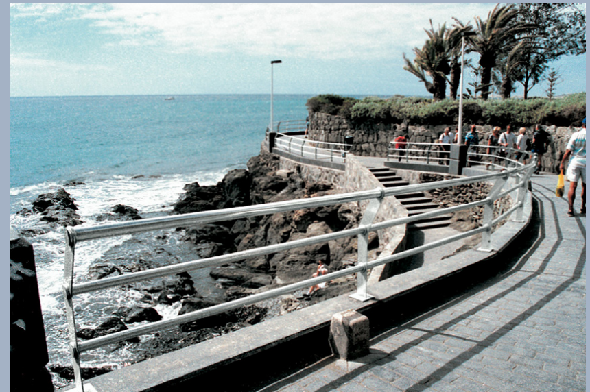
Canary Island railing, 2205 stainless steel
